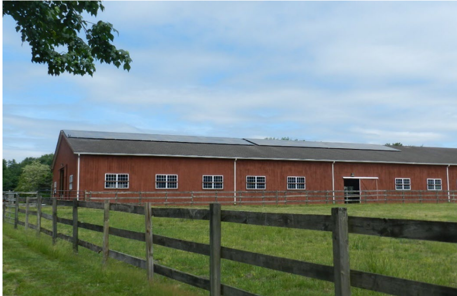
Rooftop solar panels on a preserved farm (Monmouth County Division of Planning)
